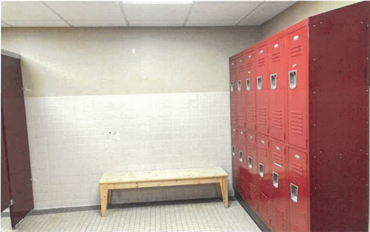
Men's Locker room including changing area and lockers
