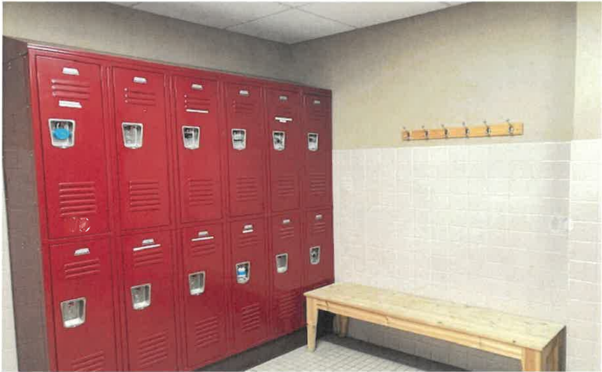
Women's Locker room including changing area and lockers
