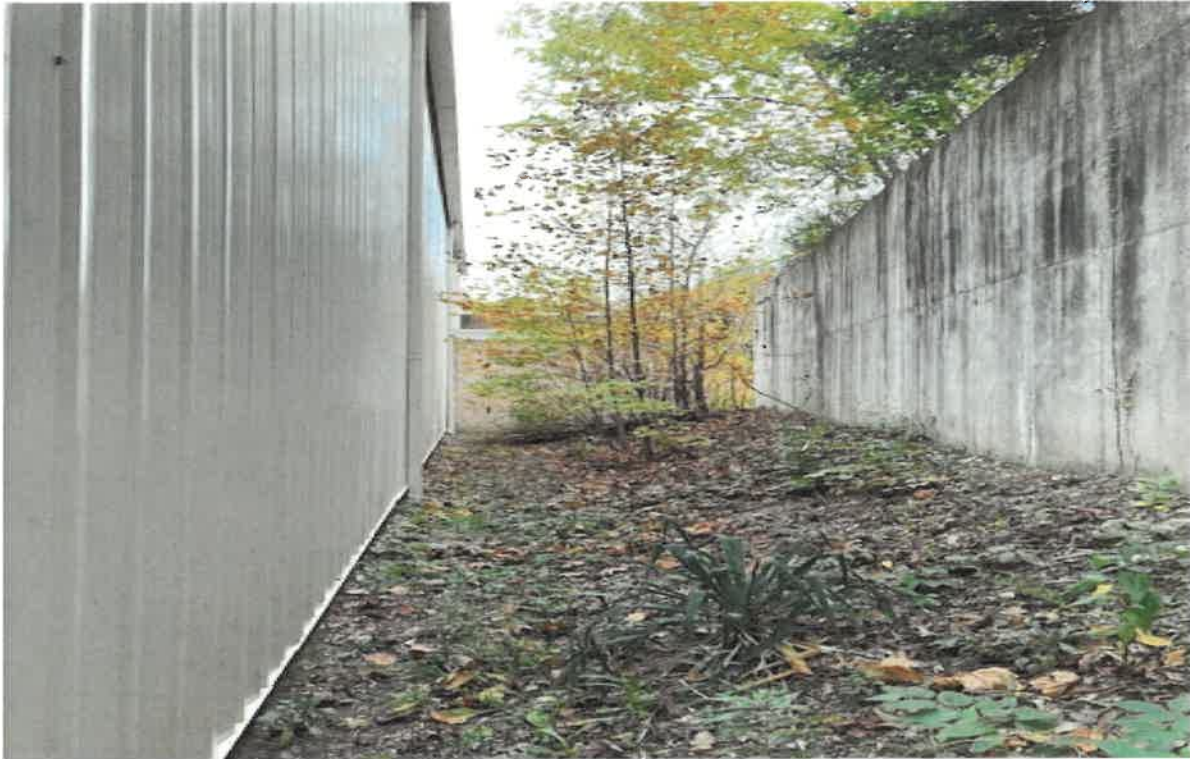
South side of property, the retaining wall with weep holes in place, along the entire span.
