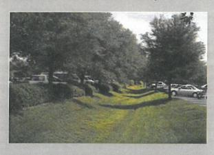
Grass Swales are designed as conveyance systems with enhanced design features to also provide a level of stormwater treatment and retention.
