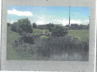
Constructed Stormwater Wetlands are shallow vegetated depressions with multiple cells of varying depths. Stormwater wetlands are not considered a runoff reduction practice, but can be used for water quality treatment and, in some cases, to meet stormwater detention requirements.
