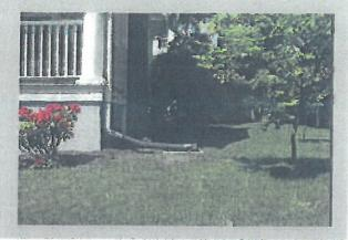
Simple Impervious Disconnection is a landscape practice that directs runoff from rooftops and other small areas of impervious surface to adjacent pervious areas as sheet flow.
