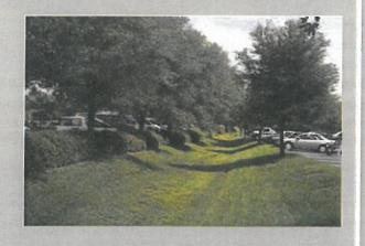
Grass Swales are designed as conveyance systems with enhanced design features to also provide a level of stormwater treatment and retention.
